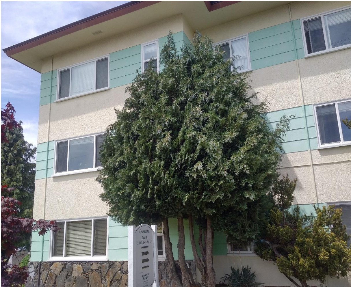
Figure 10 - The Location of the Original Victoria Ice Arena, Photographed in 2017
