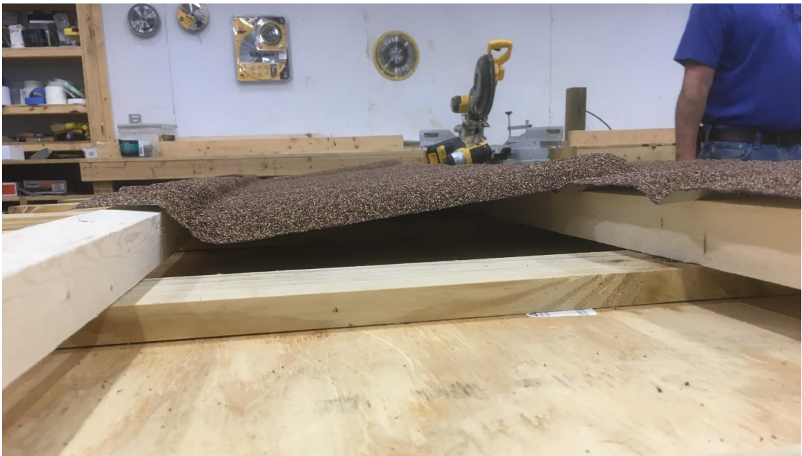
Figure 3.13: Photograph of metal panels being installed on to battens, demonstrating nailing locations, and cavity details.
