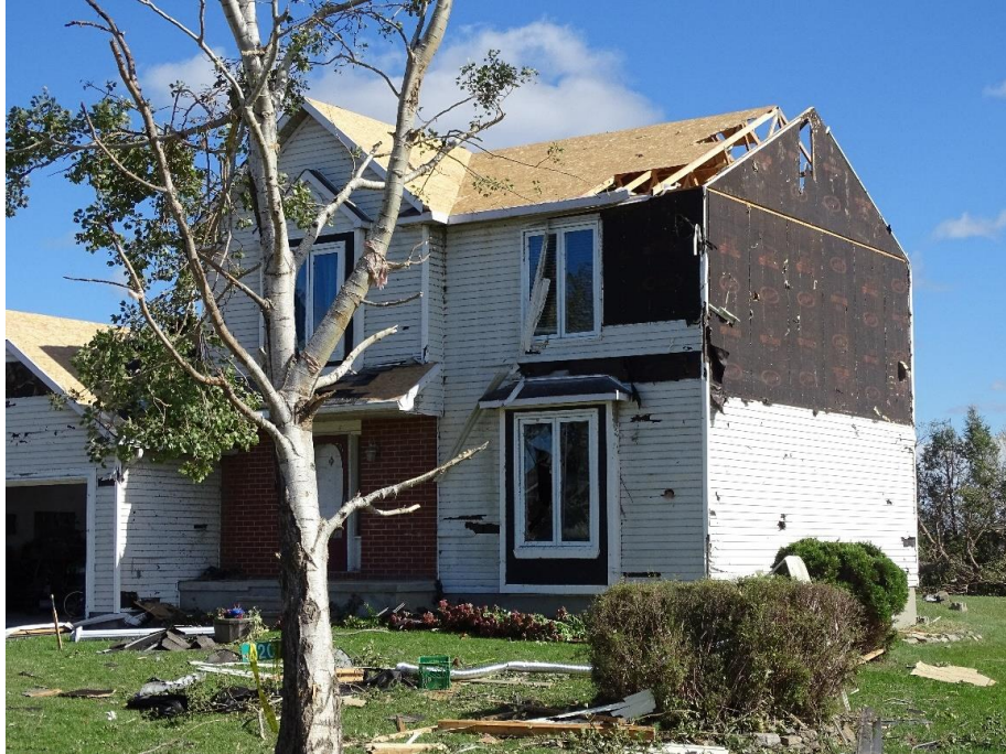
Figure 1.1: Photograph of a two-story residential building with significant component and cladding failure in Dunrobin, Ontario taken on September 21, 2018.
