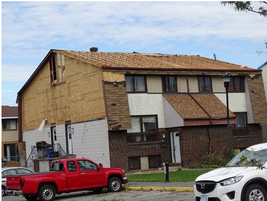
Figure 1.1: Photograph of a two-story residential building with significant component and cladding failure in Dunrobin, Ontario taken on September 21, 2018.
