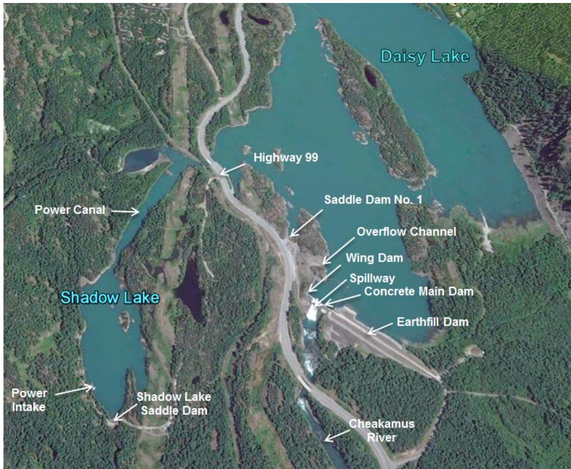
Figure 4-3: Cheakamus dam site overview
