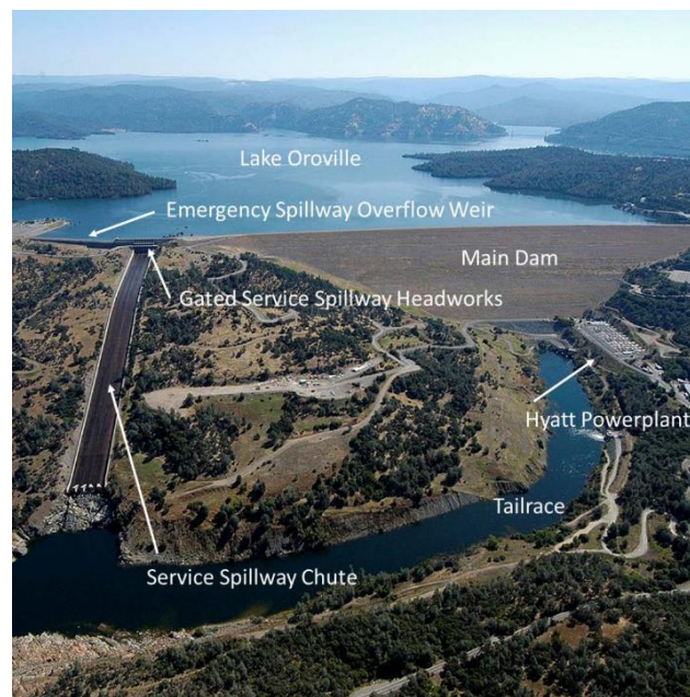
Figure 1-11: Overview of the Oroville Dam (France et al. 2018)
