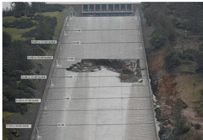
Figure 1-12: Oroville spillway chute damage (France et al. 2018)
