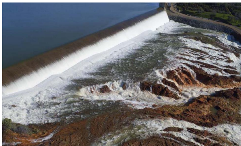
Figure 1-12: Oroville spillway chute damage (France et al. 2018)
