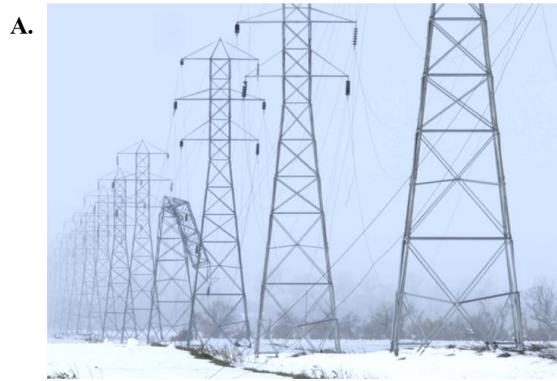
Figure 1-3: (A) Failure of one TL tower within the line. (B) Close-up image of a failed transmission line tower within a TL. “Manitoba Hydro, 2019”.
