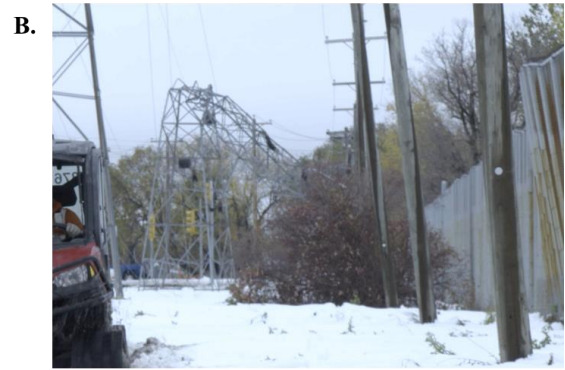
Figure 1-3: (A) Failure of one TL tower within the line. (B) Close-up image of a failed transmission line tower within a TL. “Manitoba Hydro, 2019”.
