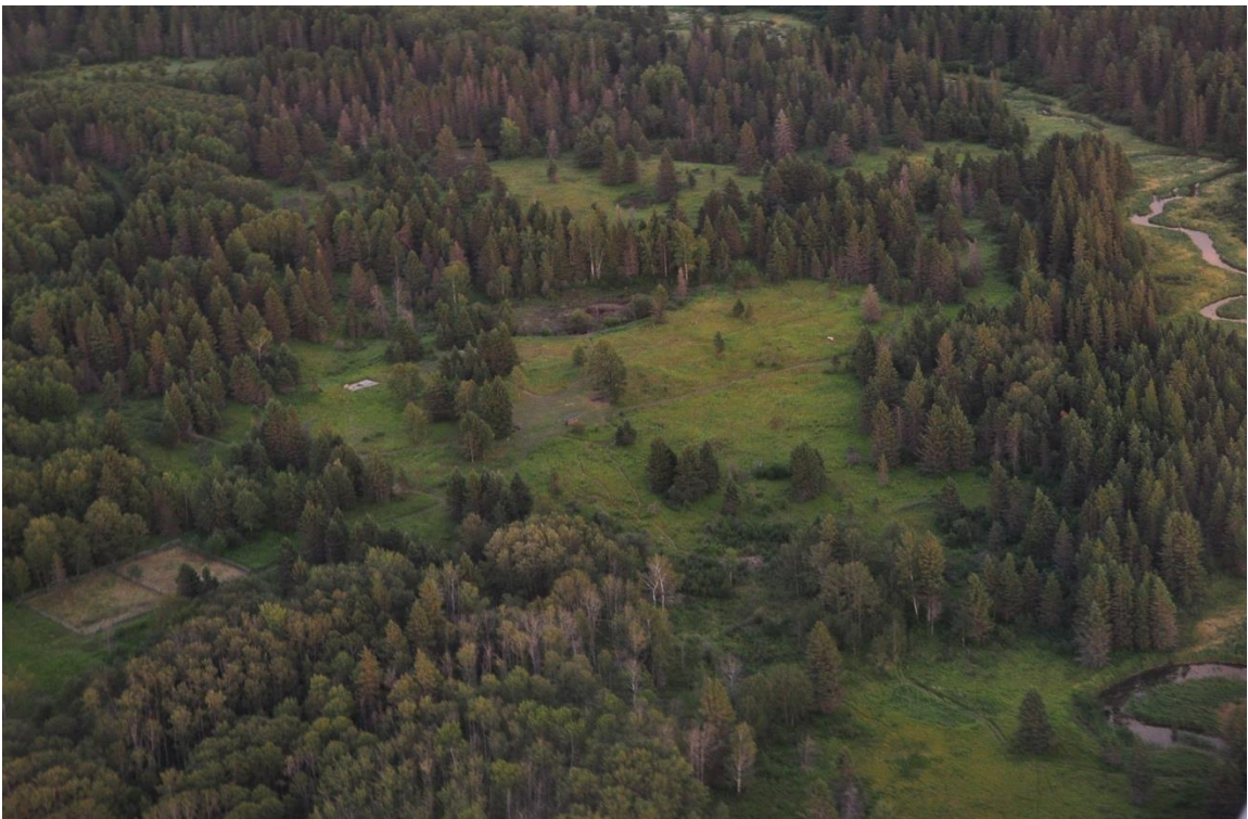
Figure 16: Aerial view of the site of the Riding Mountain Park Labour Project, 2011. The camp occupied the clearing in the centre of this photograph but the forest has reclaimed much of the site. Foundations and earthen berms are some of the only remaining signs that 440 German POWs lived and worked in the park. Author's Photo.
