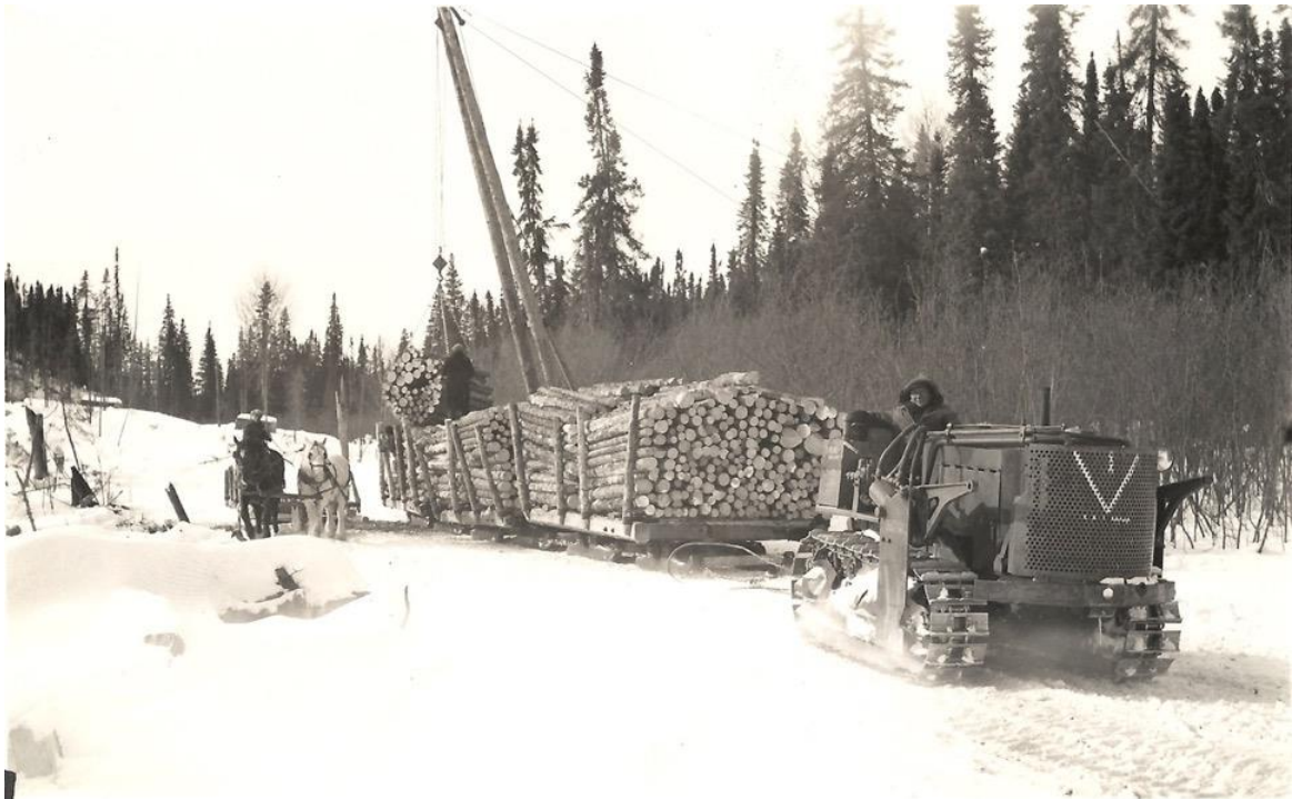
Figure 34: Hauling operations at one of Abitibi's Minataree camps. Here, a small horse-drawn load is transferred to a tractor-drawn sleigh by a log jammer (crane). The tractor would then tow the sleighs to a nearby lake or river and dump the logs on the ice. Author's Collection.
