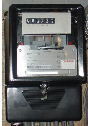
Figure 2.2: Three-phase electromechanical induction meter, metering 100 A 240/415 V supply. Horizontal Aluminum rotor disc is visible in center of the meter.(online at bit.ly/2QH1i1i )
