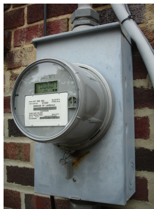
Figure 2.3: Newer retrofitted U.S. domestic digital electricity meter Elster REX with 900MHz mesh network topology for automatic meter reading and (EnergyAxis) time-of-use metering.(online at bit.ly/2QH1i1i )
