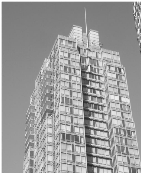
Figure 1-2: The façade of this condominium tower is covered with low thermal resistance and high solar gain curtain wall (Straube, 2012)
