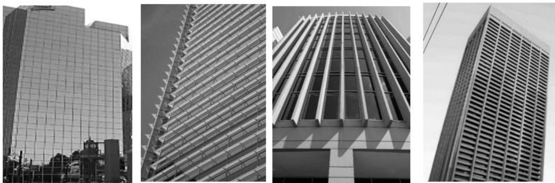
Figure 1-4: A case study on high-rise buildings model a) without shading b) horizontal shading c) vertical shading and d) egg-crate shading
