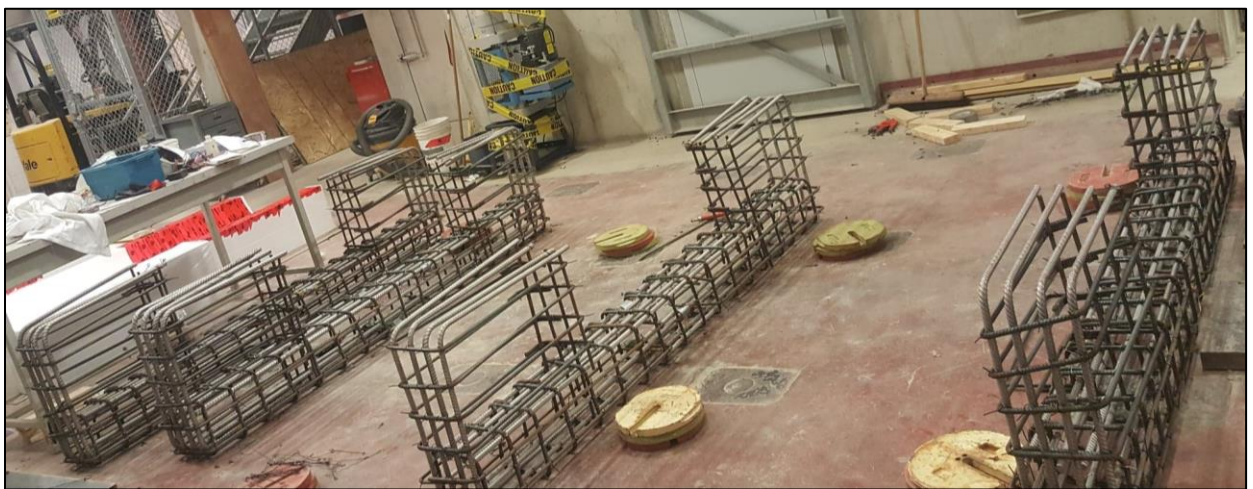
Figure 4.5: Steel Cages of the Tested Columns
