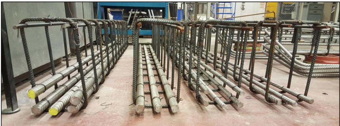
(a) Steel Cages of the Considered Beams
