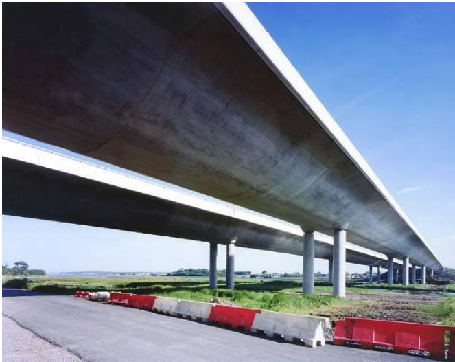
(a) Bridge photo
