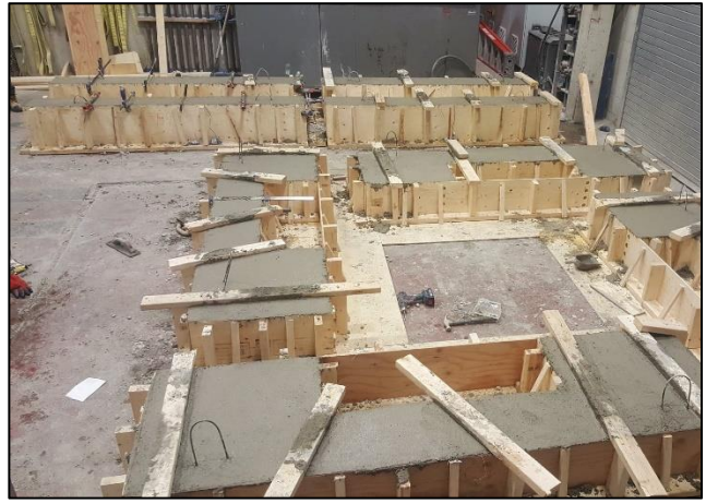
(c) Concrete Poured into Formworks
