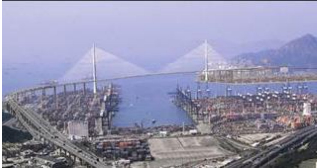
Figure 2.3: Stonecutters Bridge, Hong Kong [12]
