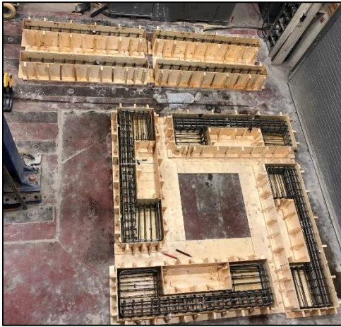
(b) Steel Cages in Formworks
