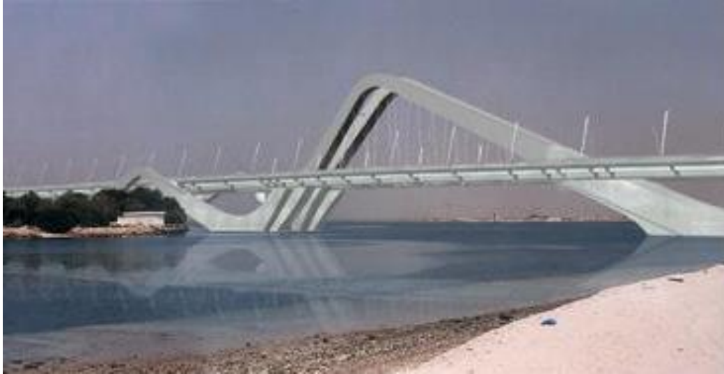
Figure 2.5: Sheik Zayed Bridge, Abu Dhabi [12]
