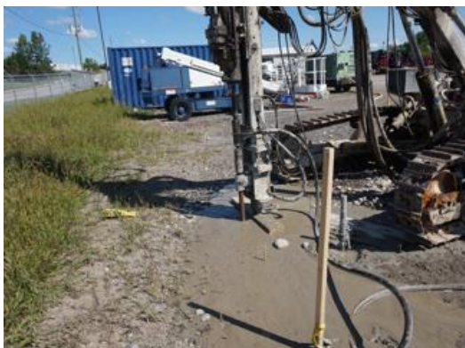
(e) Finish drilling
