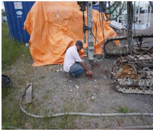
(a) Setting micropiles location
