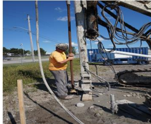
(b) Attaching the hollow bar to the driller
