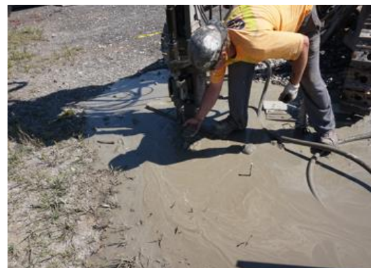
(f) Pressurizing the competent grout
