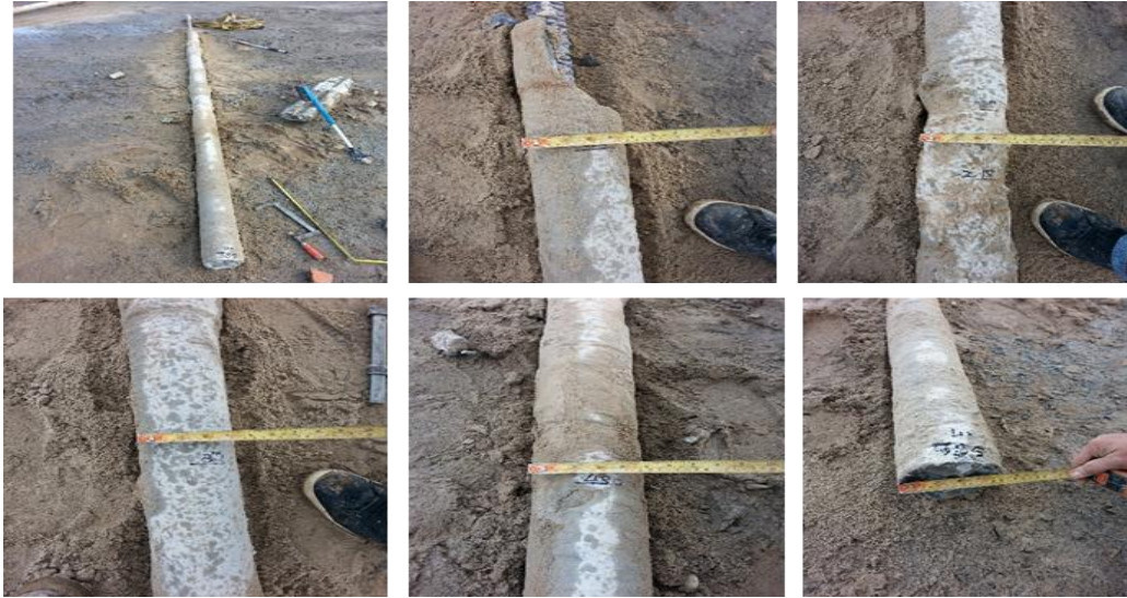
Figure 5-11 Exhumed micropile MP3 and diameter measurement along the depth
