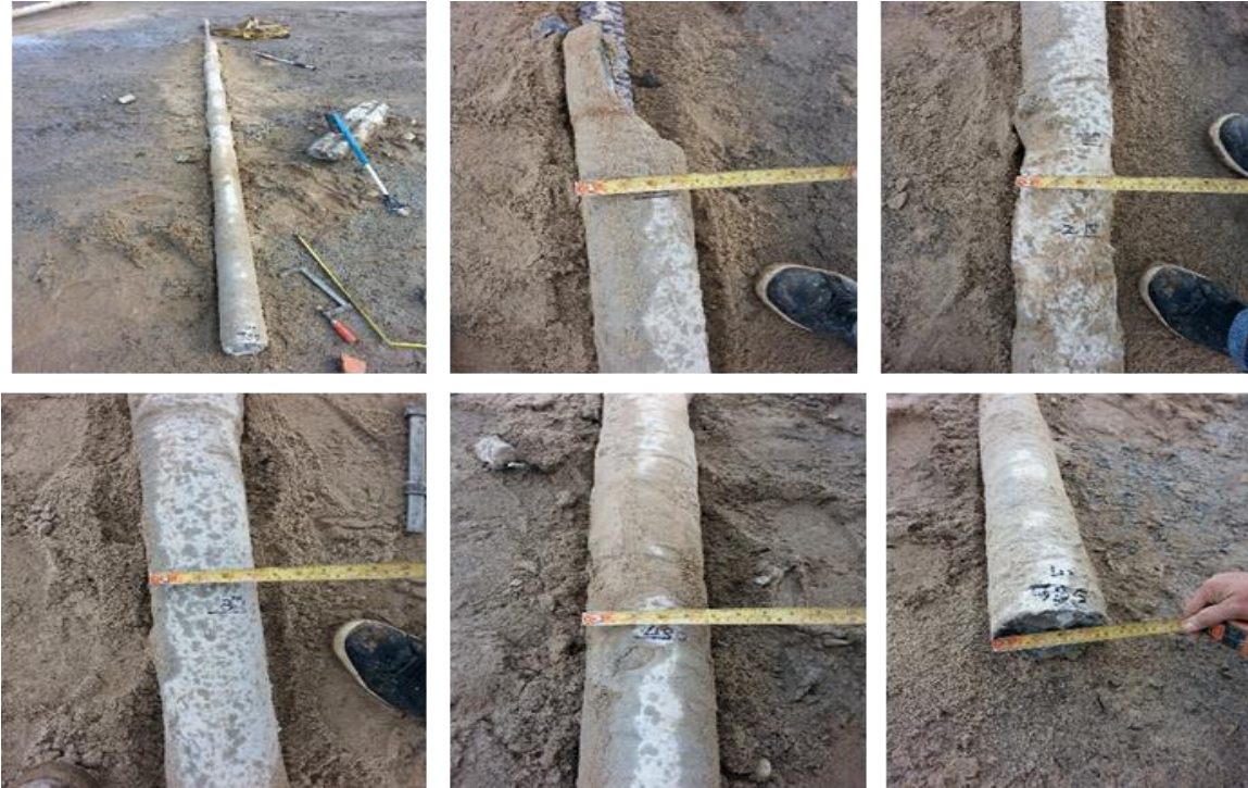
Figure 3-10 Exhumed micropiles MP3 and diameter measurement along the depth
