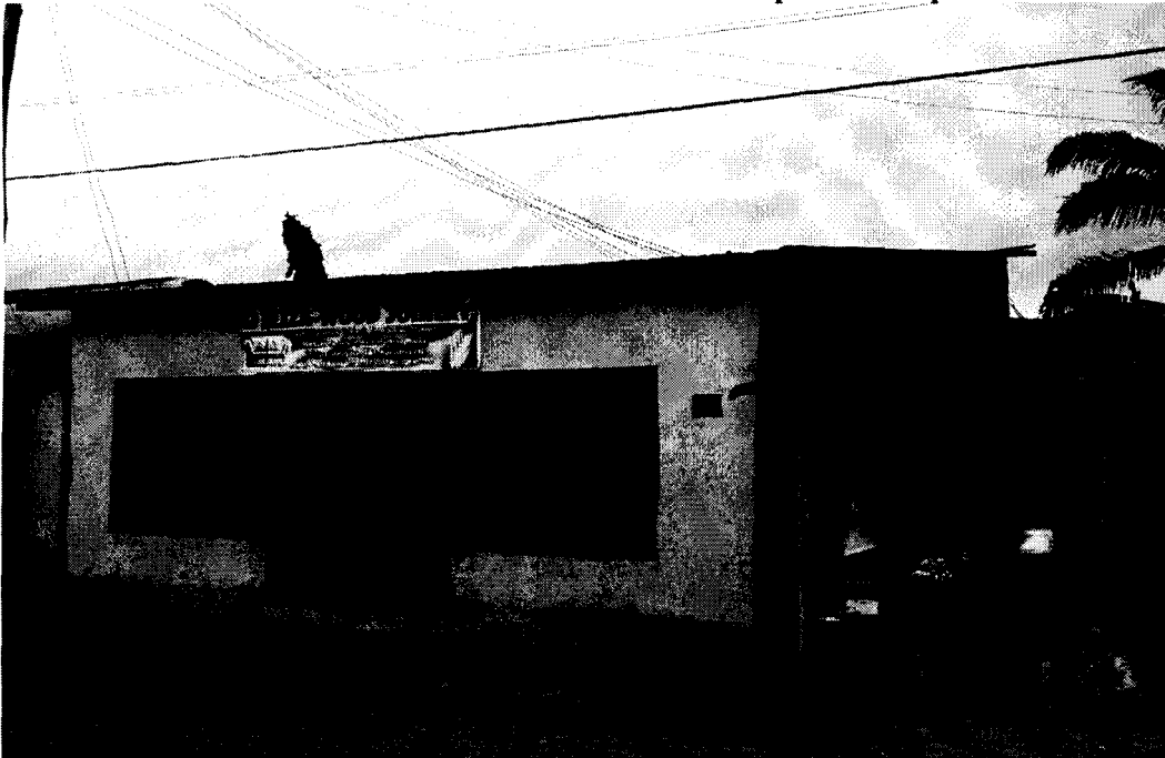
Plate 4.4: House extended to roadside and converted in a shop and workspace
