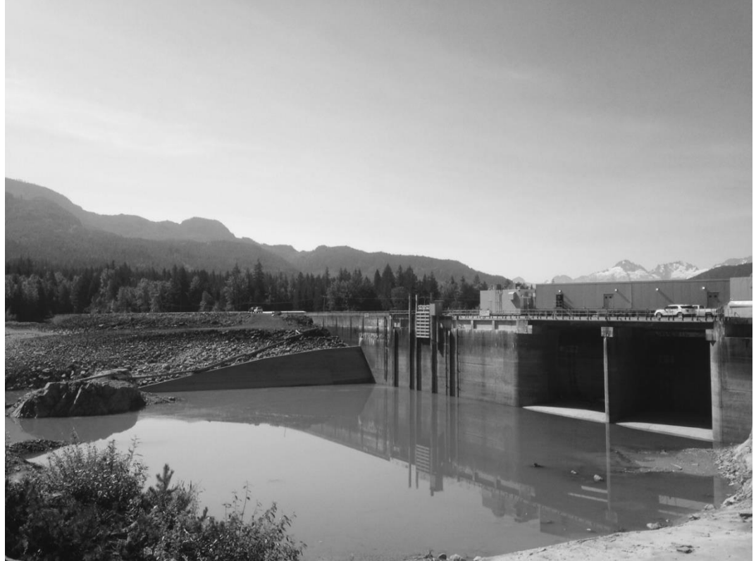
Figure 10: Cheakamus Dam (photo taken by Ryan Weise on August 11, 2015)
