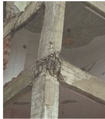
(b) Close up view of the third-level BCJ
