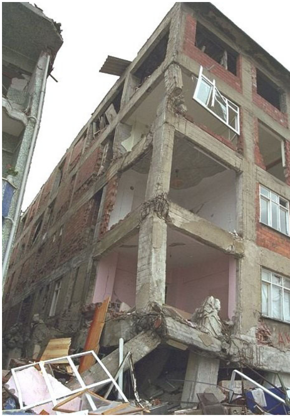
(a) Full view of the building
