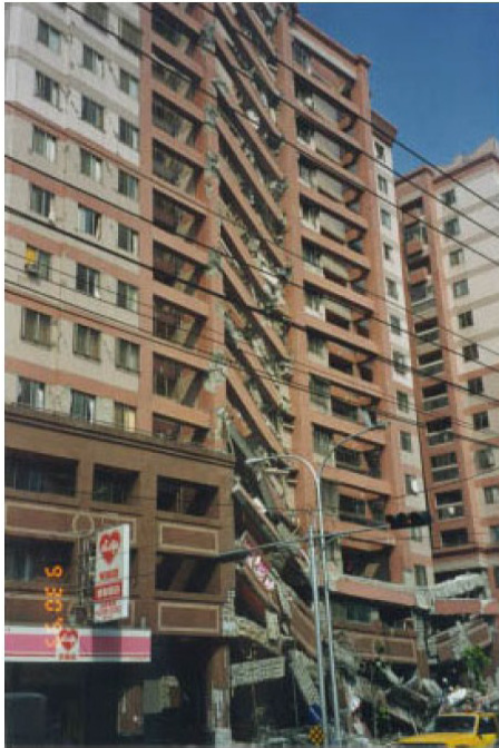
(a) Full view of the building
