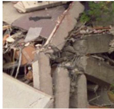
(b) Close up view of the failed BCJs
