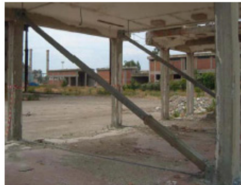
Fig. 2-14: Retrofitting of a two storey RC frame using SMAs (Dolce et al. 2004)
