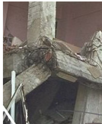
(c) Close up view of the second-level BCJ
