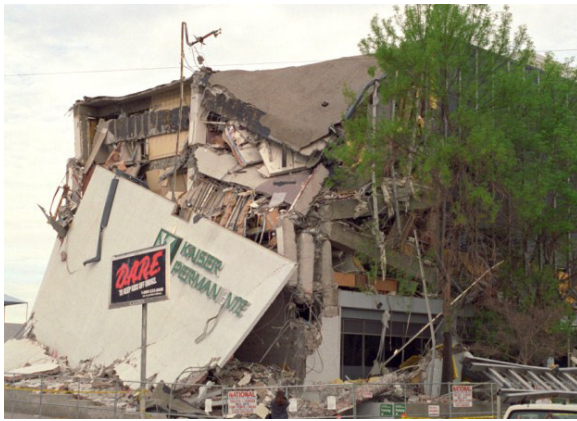
(a) Full view of the building
