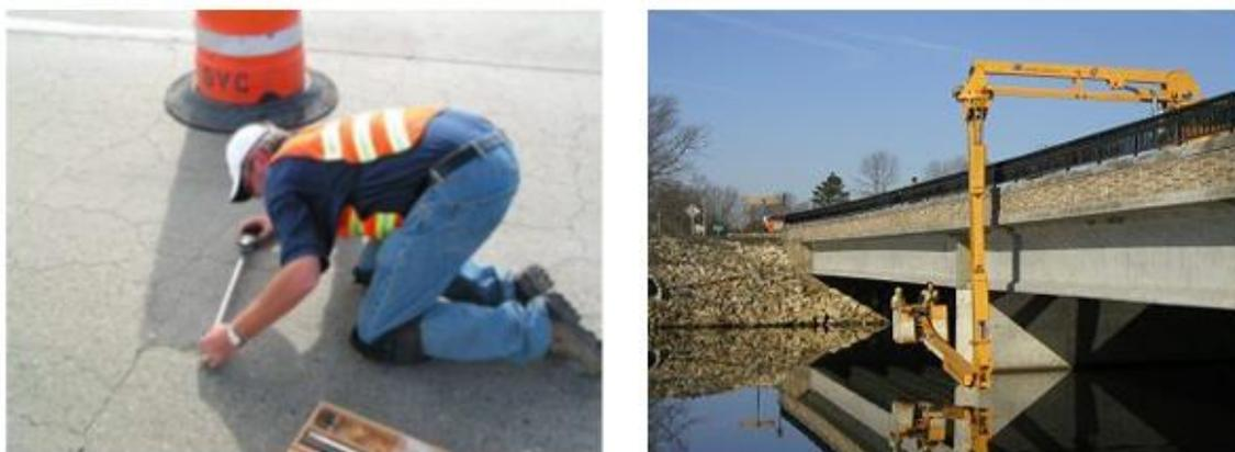
**Figure 2-4: Visual inspection of concrete bridge decks and soffits (Gucunski *et al.*, 2013).**
