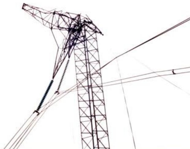
**Figure 1-4 Broken cross-arm due to downburst event “Aboshosha et al. (2016a)”**
