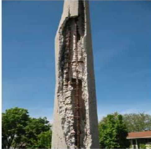
**Fig. 1-3** Longitudinal cracking, corrosion and spalling caused by differential shrinkage and segregation of concrete mix (Kuebler 2008)
