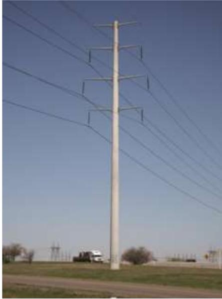
(a) Cantilever concrete pole
