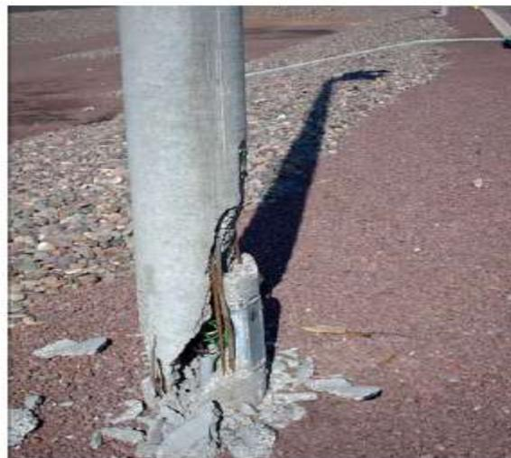
**Fig. 1-2** shear failure of the pole due to a vehicle impact (Kuebler 2008)
