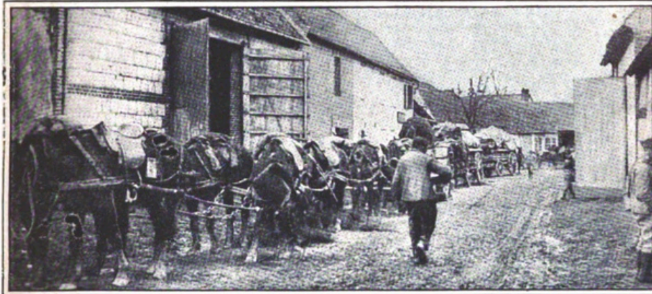
THE TWENTIETH CENTURY CARAVAN
