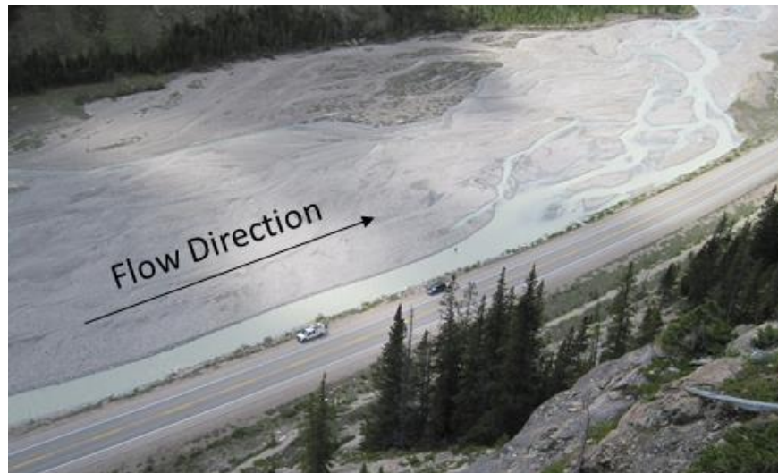
Figure 7.7: The current braided configuration of the Sunwapta River where the primary channel is seen to lie against the highway, reducing the rate of planform change.
