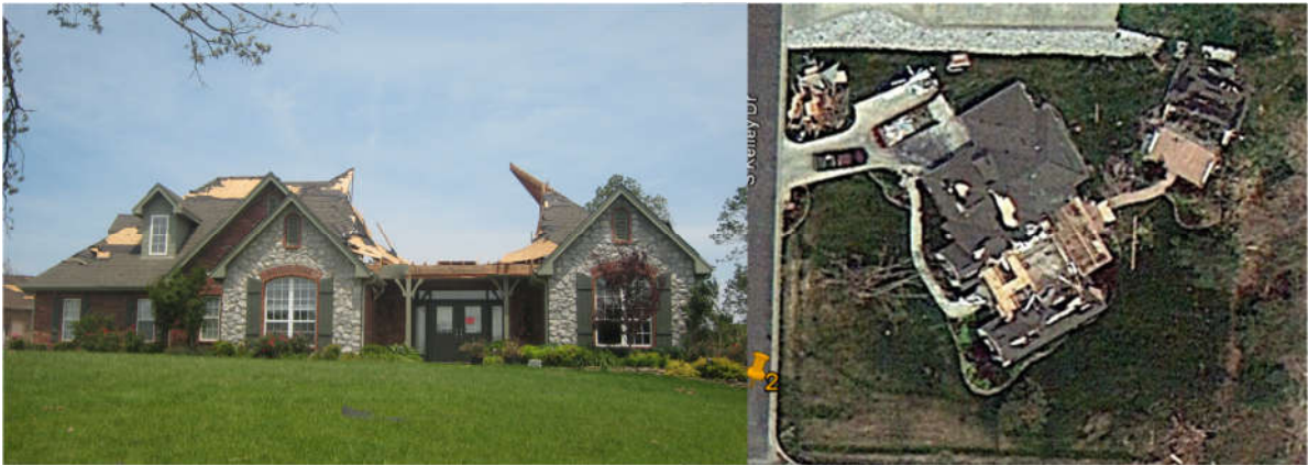
Figure 1-7: Example of typical hip roof configuration in Region 1, with an aerial photo showing the footprint of the partial failure on the right-hand side of the figure (Image provided by Dr. David Prevatt, Google Earth)
