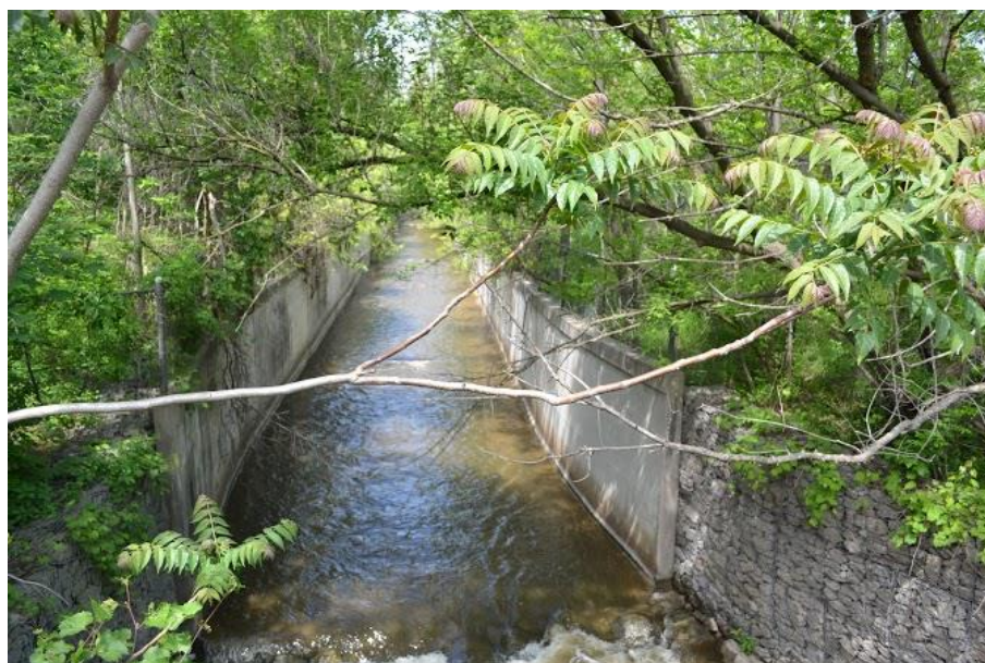
Figure 5: Bank Stabilizing Structures in Spencer Creek
