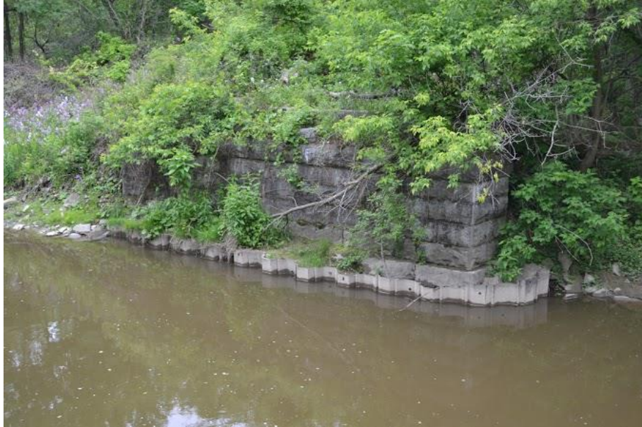
Figure 50: Spencer Creek Bank Stabilization Structure
