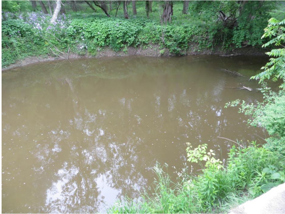
Figure 46: Spencer Creek downstream showing bank erosion
