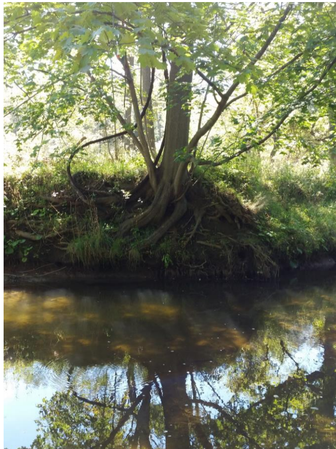
Figure 51: Spencer Creek Exposed Tree Roots
