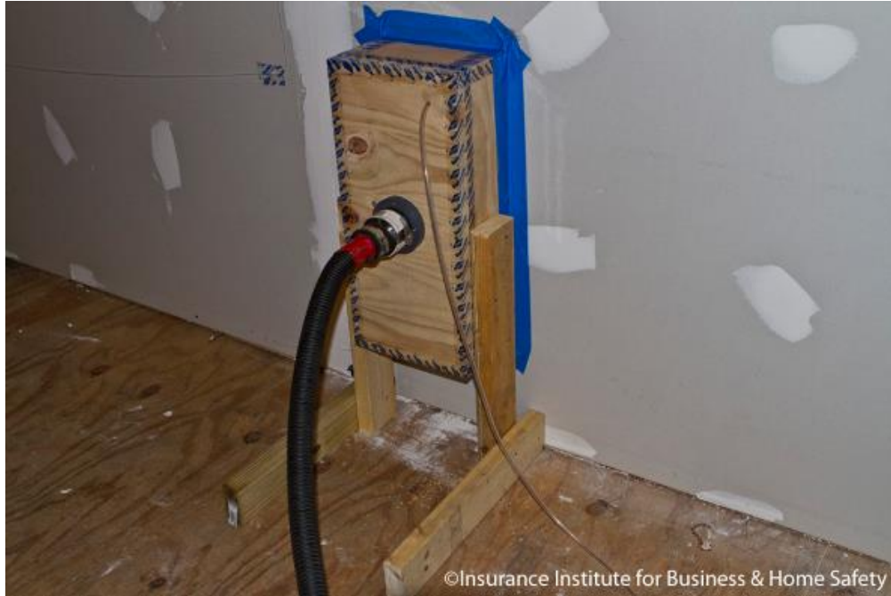
Figure 84: Photo of airbox mounted over electrical outlet and ready for testing.
