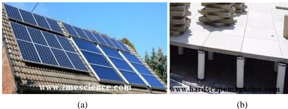
Figure 1-3: Example of double-layer systems (a) Solar panel array on a sloped roof (b) Loose-laid roof pavers
