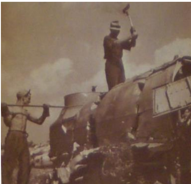
Photo 11 Workers at St. Johns, Quebec scrap old damaged aircraft that cannot be sold any other way. Source: LAC, RG101, Vol. 1, File: R-1-1-9 History of War Assets Corporation Ltd. and War Assets Corporation, Newspaper Clippings, The Standard , 15 September 1945, 8.
