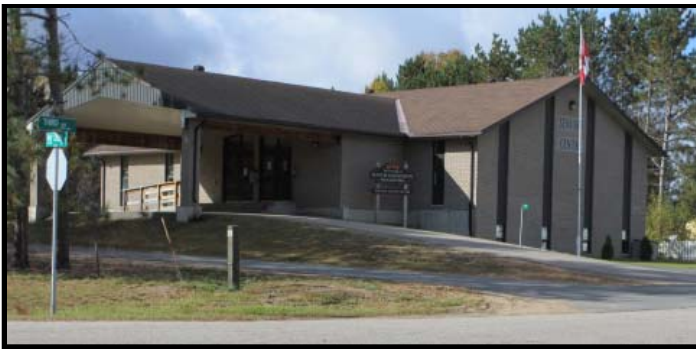
Figure 58: Seniors Centre, Township of South Algonquin Offices
