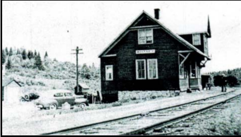
Figure 52: Whitney Railway Station
