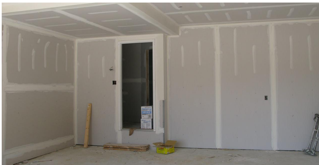
Figure 1.1: Typical Application of Gypsum-Board Sheathing
