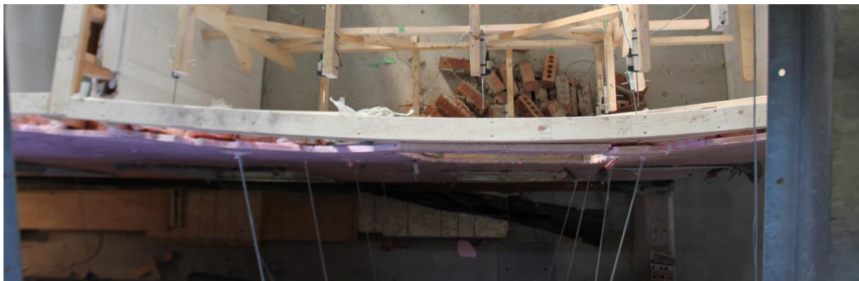
Figure 6.8 - The top plate of exterior wall A1-D1, immediately before failure.
