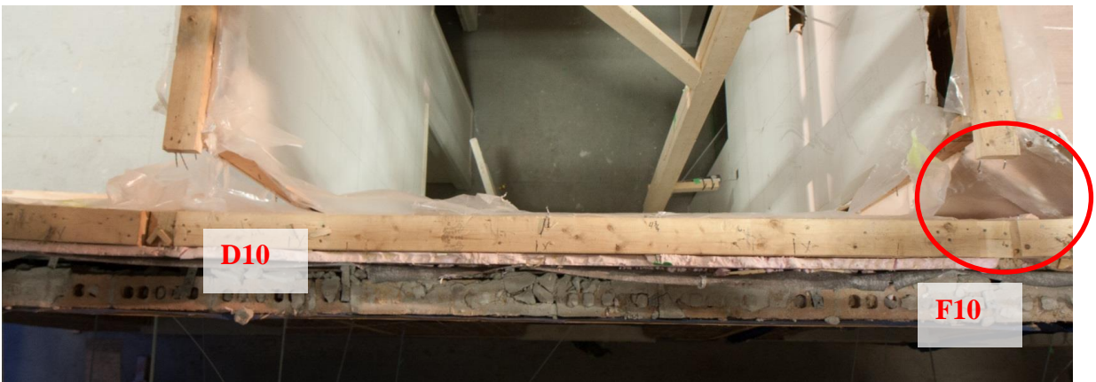
Figure 5.4 - Wall D10 - F10 after both joints have failed.
