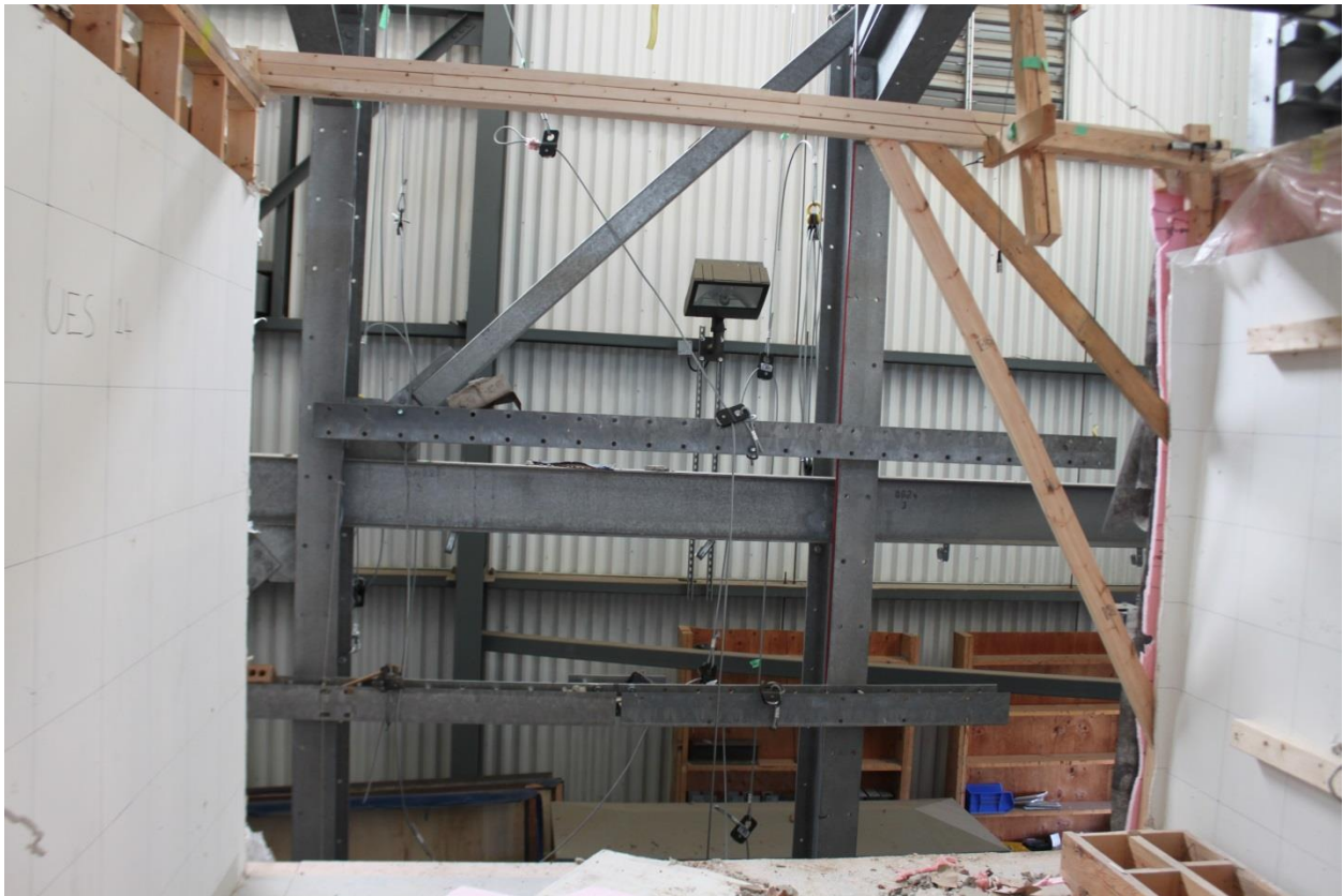
Figure J1 - The false top plate installed at A10-E10 to increase the stiffness of wall A1-J1.
