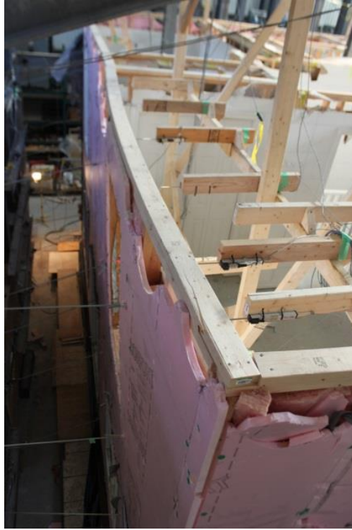
Figure 6.7 – Exterior wall looking from A1 – foreground and D1 – background.
