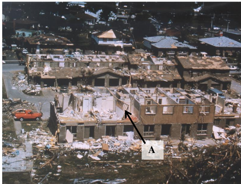
Figure 1.3 - Tornado damage in Barrie, Ontario 1985 (from Davenport and Kopp, 2002).
