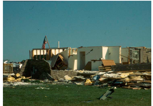
Figure 1.2- A reference for degree of damage seven (from Texas Tech University, 2006).
