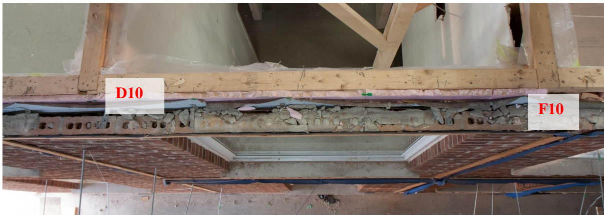
Figure 5.1 - Wall D10 - F10 before loading.
