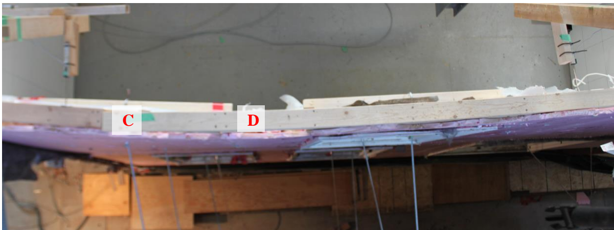
Figure 6.4 - The North East wall prior to failure E1 – J1.
