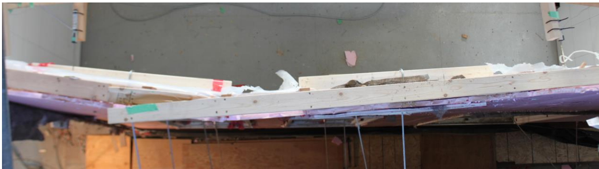
Figure 4.6 - Plan view of wall E1-J1 after catastrophic failure.
