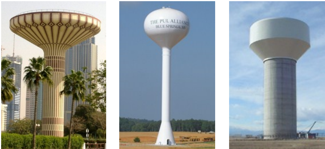
Figure 1-1 Different Configurations of Elevated Tanks
