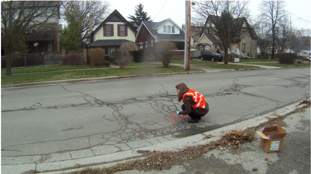
Road Work . Documentation of process. William St. 2012
