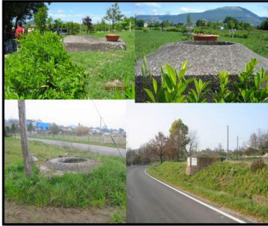
A series of German tobruks located in Cassino, Italy on the Hitler Line. The concrete, about four feet into the ground below what is visible, is impossible to move. The civilians incorporate it into their landscape. The top one has become a stand for outdoor plants. (Photos courtesy of Raymond Gallant and Ashley Ferguson, study tour participants, The Second World War in Italy , 2012 and Eric McGeer, co-author of The Canadian Battlefields in Italy guidebook)
