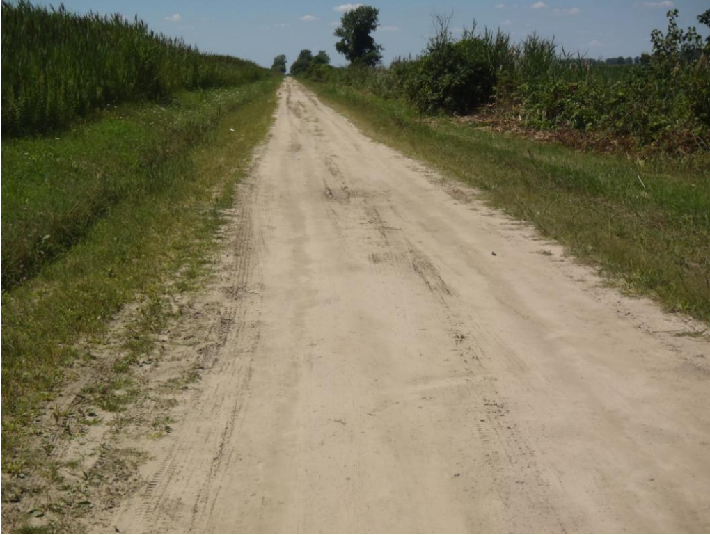
Figure A2.19 Roads on the marsh dikes are made of compacted soil.
