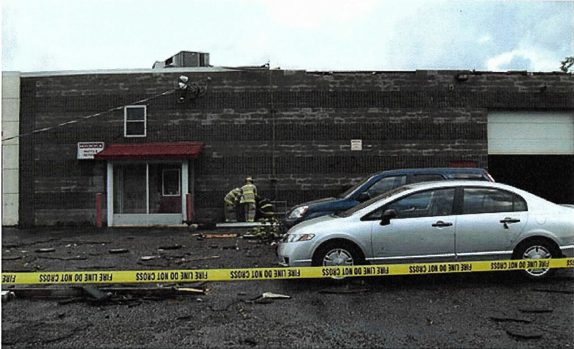
Police lines surround a damaged building in Midland. Submitted by thefoxman.
