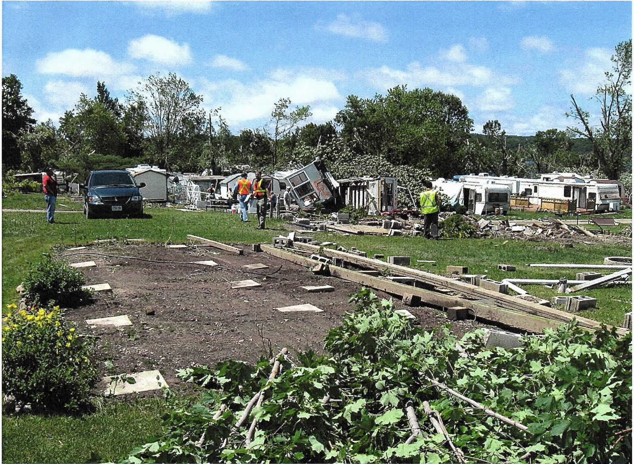
Figure 6: Smith Trailer Park located in Midland. Picture looking southwestward showing the location of a 40ft trailer that had been uplifted and displaced 28m to the north. Trailers that had been uplifted and thrown more than several tens of meters were
