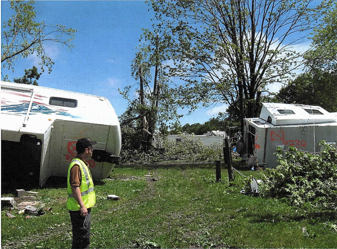
Figure 4: Smith Trailer Park located in Midland. Picture looking eastward showing two full sized 35ft trailers rolled on their side and numerous surrounding trees sheared off at the top. There was no evidence of anchoring to the ground in most trailers within the park.
