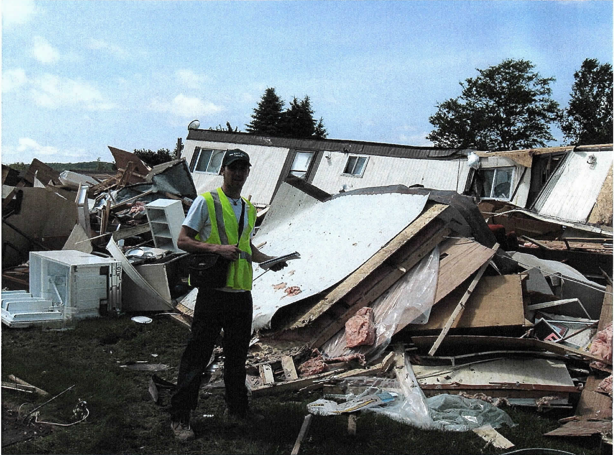
Figure 7: Smith Trailer Park located in Midland. Picture looking southwestward showing a permanent modulated home that had collapsed and interior items uplifted. Seven permanent modular homes were severely damaged. Attached to waypoint 19.
