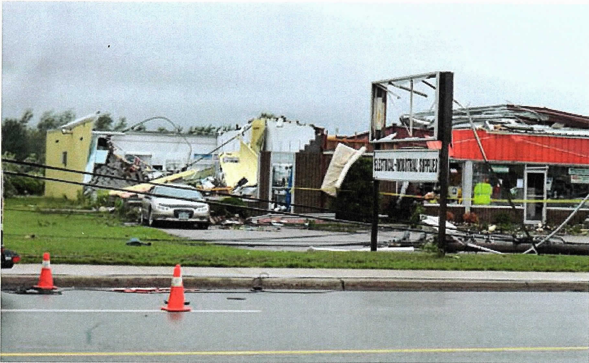
Local businesses suffered damaged exteriors. (Submitted by Genessee Walker-Scace)
