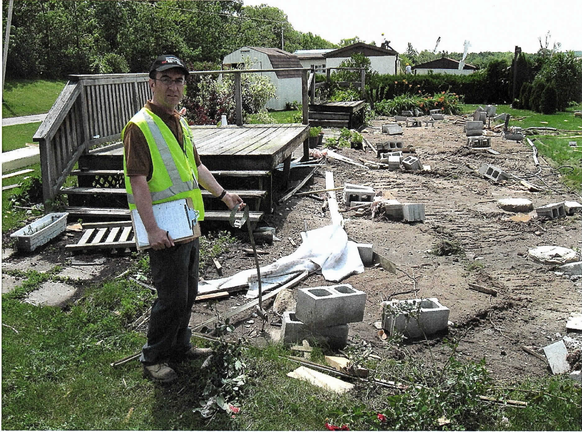
Figure 13: The site of origin for the modular home that was entirely uplifted and relocated on Vics Rd. Picture looking southwest showing the steel metal anchors and hooks that failed to secure the modular home to the ground. Attached to waypoint 19.
