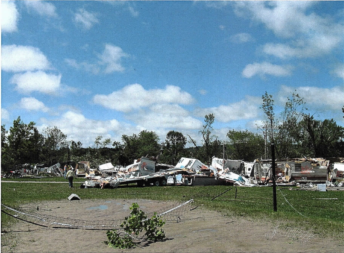
Figure 5: Smith Trailer Park located in Midland. Picture looking westward showing the scattered debris and destroyed trailers at the southwestern portion of the park where the mobile homes were situated. Attached to waypoint 18.
