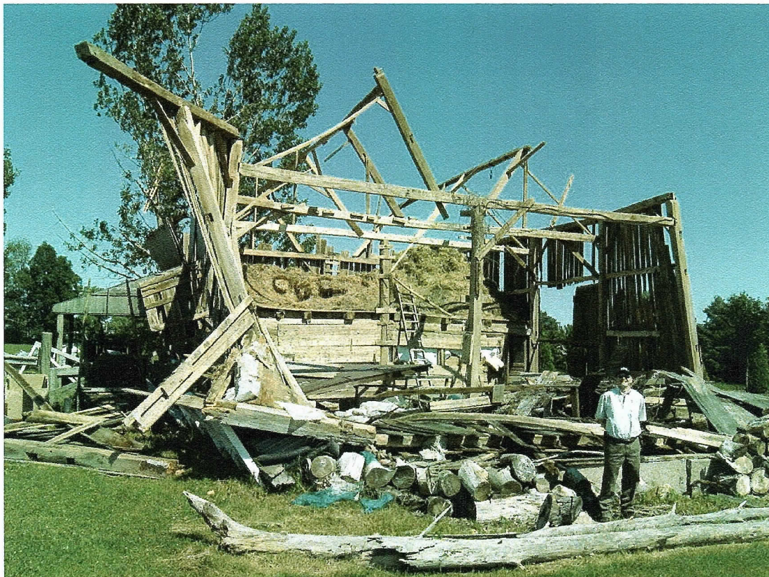
Looking East Lat/Long - 42.0076N, 82.5452W Barn on the west side showing most extensive damage to the structure, showing collapsed west wall and roof removed
