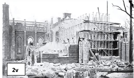
Demolition of Gore Hall, 1913; note the five tiers of self-supporting bookstacks. (Public domain; from Snead & Co’s Library Planning.)
