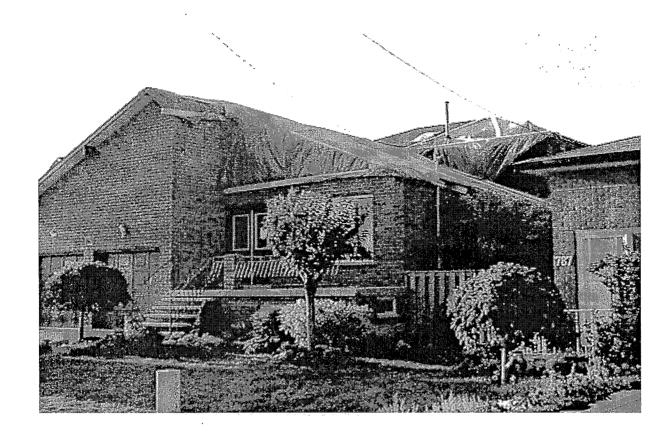
The large area of missing roof and questions about the structural integrity of the remaining roof resulted in the family being forced to move out. A neighbour reported seeing swirling debris at this location. This house had gotten much media attention (see Appendix B) and is on the north side of Stone Church, meaning the tornado had now tracked NE from the house that had its siding removed.
