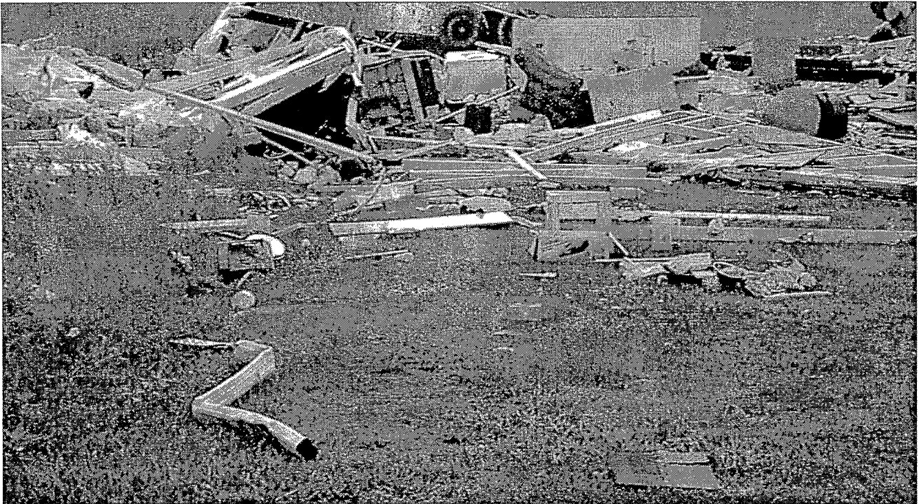
Facing W, mobile home base upside down and roof, walls and contents scattered downwind.
