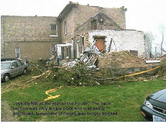
Looking WNW at the rear of the house. Most brick from the wall fell directly downwards, hole in the wall is to the upper right of the photo. (Side of the house facing East)
