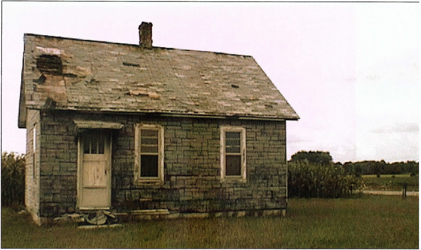
Shack with shingle damage facing NNE. The tornado moved over the shack and into the bean fields shown at the right side of the photograph.
