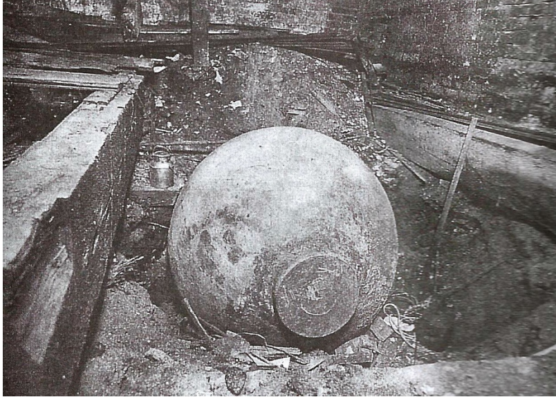
Fig. 6 After Keely and Moore died, Moore's son Clarence hired workers and investigators to dismantle Keely's workshop. They discovered a large cast-iron sphere concealed under the floor: a tank for the compressed air that Scientific American said must have powered all of Keely's inventions. (Source: "Investigations at the Keely Laboratory," Scientific American , February 4, 1899, p. 72.)
