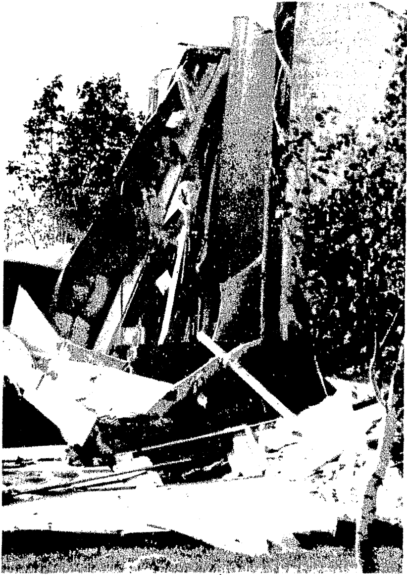
One lone wall was all that remained of the devastated home,
