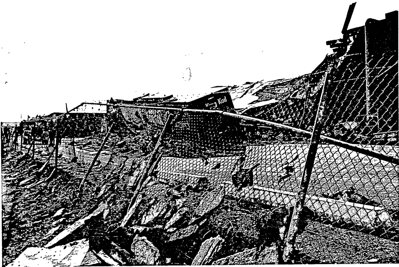
Damage to the Bedford Bedding and Upholstery Ltd North wall of factory collapsed onto parked trailer
