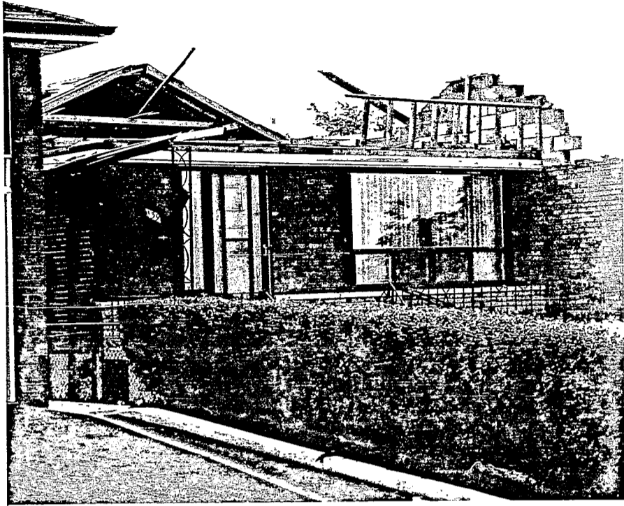
139 Honeywood - roof removed by storm
