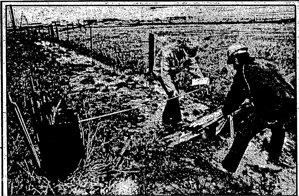
After a pole snapped on Weston Rd. near Hwy. 7, Consumers' Gas men mark gas lines so they aren't hit when a new pole goes in.
