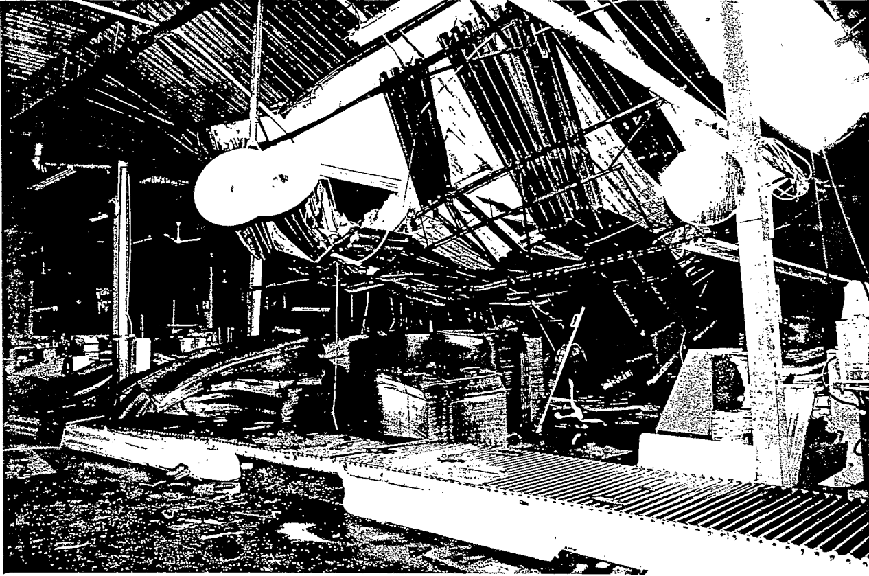
Location 1 - KRUGER PAPER CO. Factory roof collapsed
