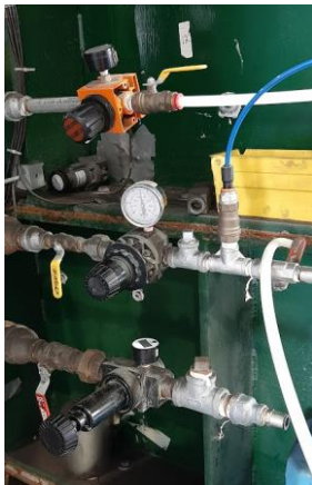
Figure 24 – The top pressure regulator is for the whole vessel, and the middle pressure regulator supplies the backflushing gas.
