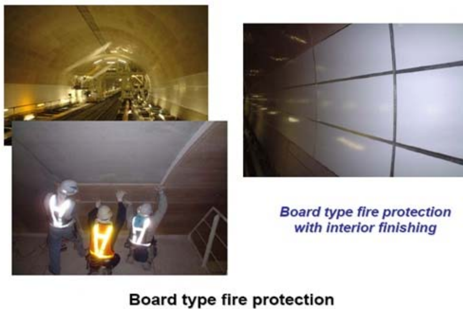
Figure 2.1 Tunnel fire protection: cladding type (board type)
