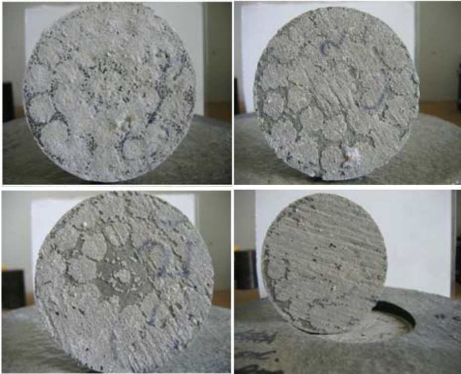
Figure 5.8 Pulled plate surfaces on concrete: a) C-1, b) C-2, c) C-3 and d) C-4
