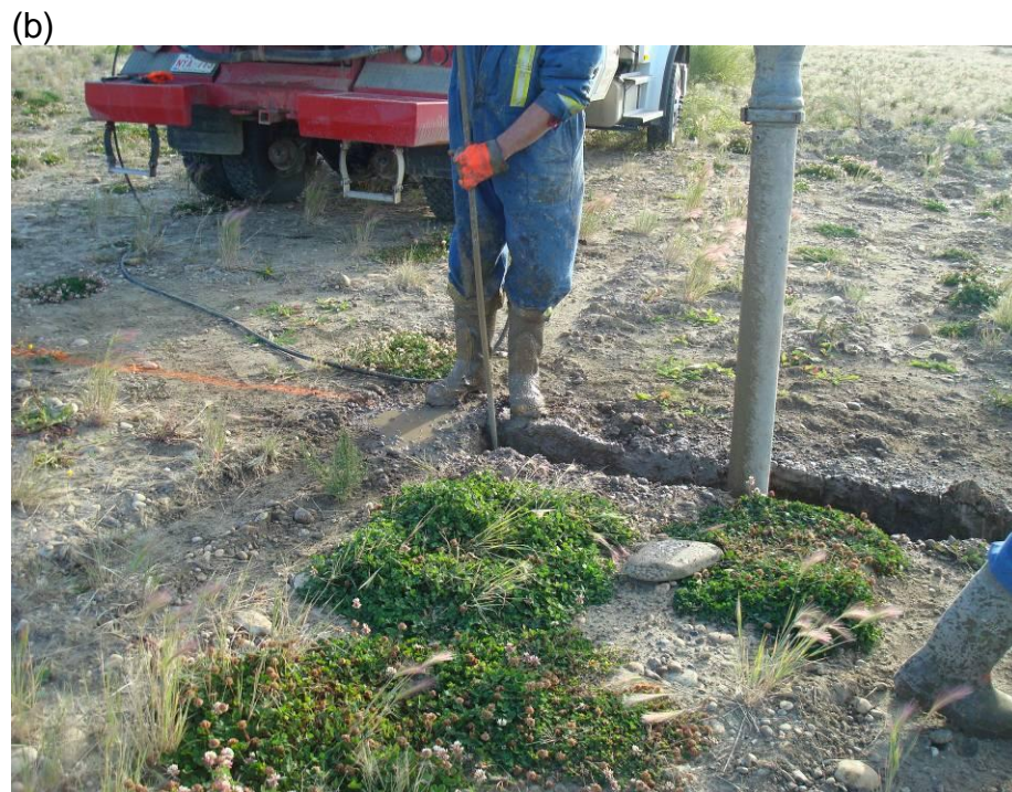
Figure 4- 3: Digging the open trench using hydro-dig technique
