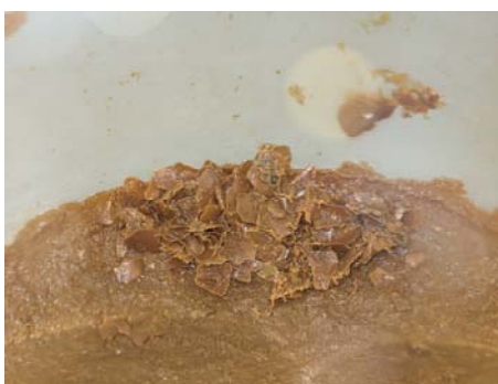
Figure 7.3 Severe mineral depositing of jarosite.
