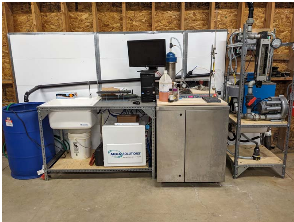
Figure E Pilot scale BioGenerator support equipment (interior).
