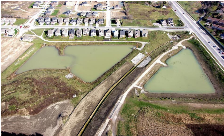
Figure 3: Fox Hollow Subdivision Stormwater Management System in London, ON (City of London, 2012)
