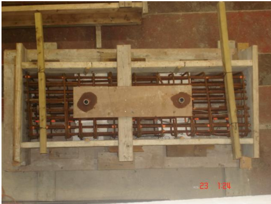
Reinforcement and formwork of the base block
