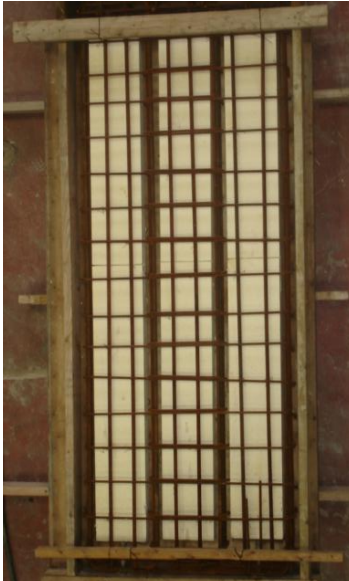
Reinforcement and formwork of the precast concrete panel
