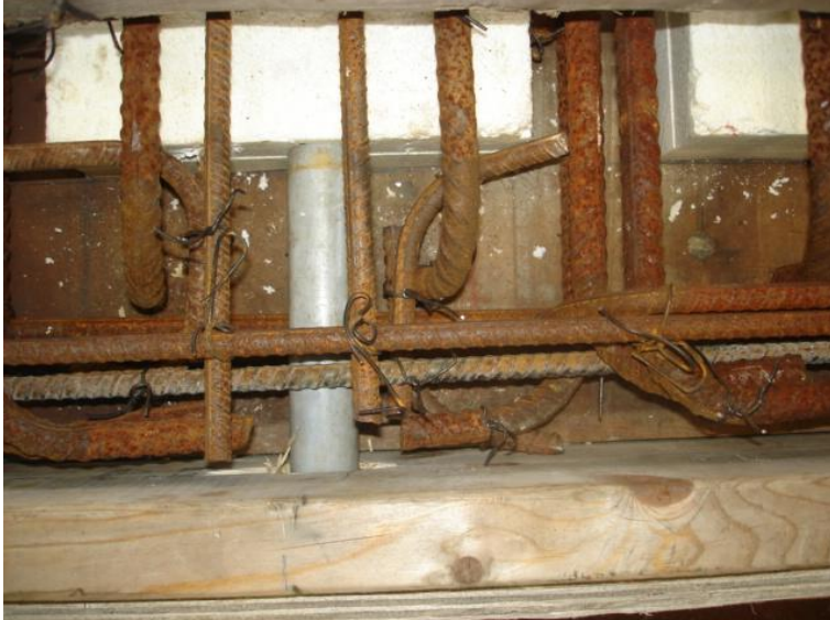
Close up to reinforcement
