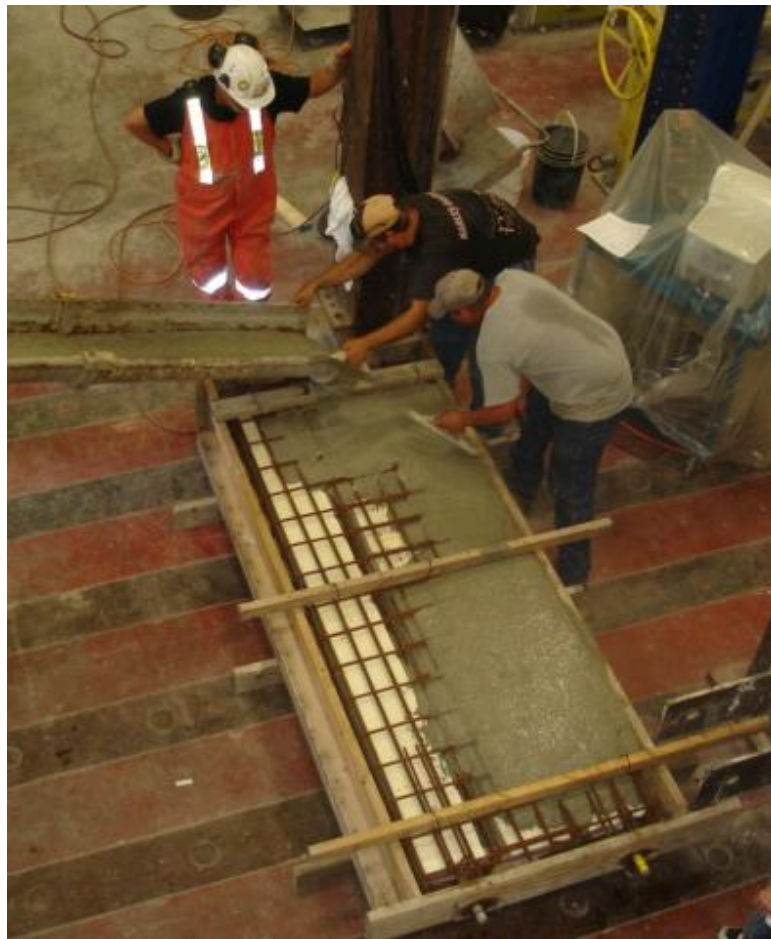
Placing concrete
