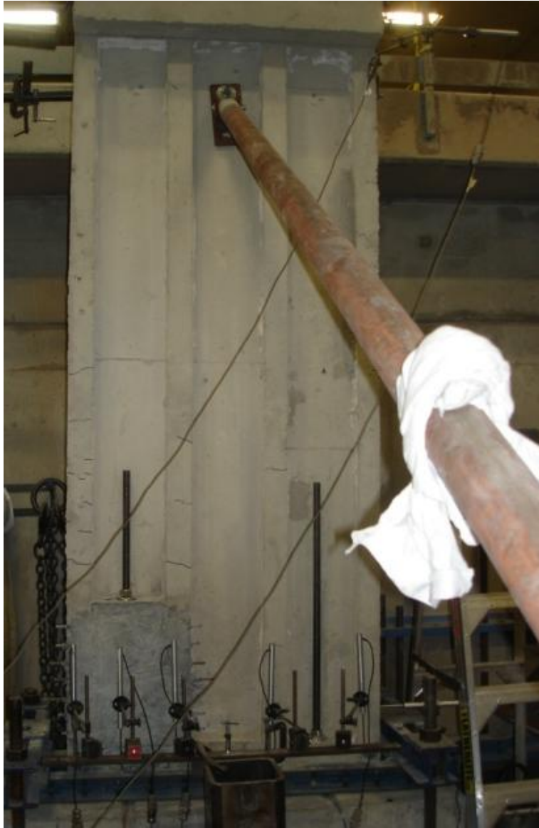
Figure 2.39: Cracks formed in the concrete panel
