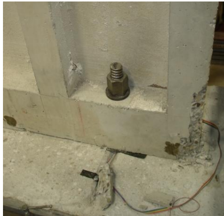
Figure 2.18: Minor cover spalling at the compression side of the joint
