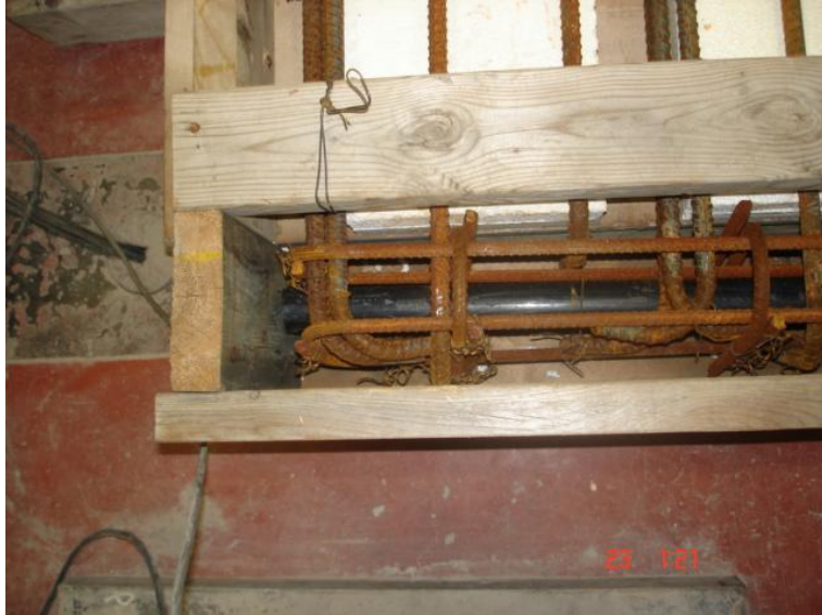
Reinforcement of the upper loading beam
