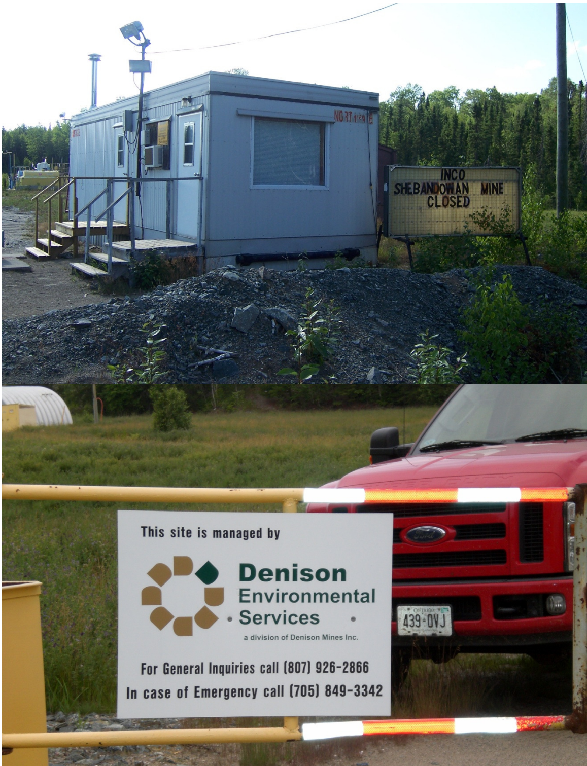
Figure IV-2 Main entrance to the Shebandowan tailings storage facility
