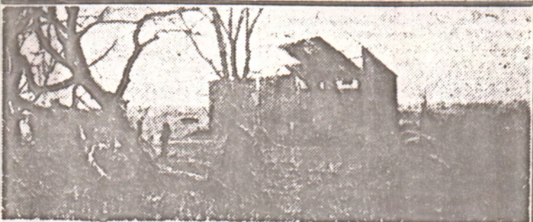
When a tiny tornado swept through the south end of Chesley last week, buildings were unroofed, wrecked and flattened, large trees uprooted, and other sections of the town sprinkled with a rain of shingles and splintered wood. A large part of the east wing of Krug brothers' furniture factory (shown above) was demolished. One section of pipe from the sprinkler system was carried 500 feet, and punctured a house window. Having finished its urban playfulness, the gale took a whirl in the neighboring countryside, repeating its tactics on barns and driving sheds. One of the shattered barns is shown below.
