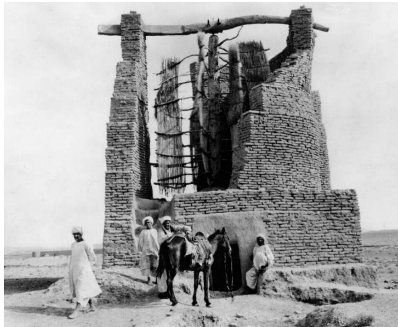
Figure 1 Vertical-axis windmill for milling grain, Afghanistan. Deutsches Museum (Hau, 2013).
