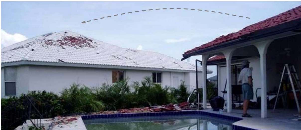
Figure 31 – Tampa, Florida. Extreme winds caused roof tile to fly and hit the neighbour’s house (photo courtesy of Tim Reinhold).
