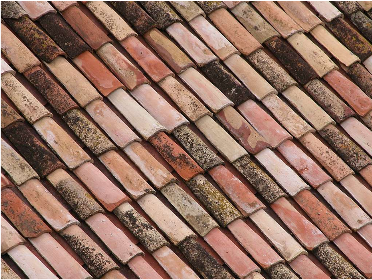
Figure 26 - Terracotta over-and-under roof tile. The geometric and material characteristics of this roof tile type follows UNI 9460 (2008). The international standard EN 14437 (CEN 2004) cannot be used to calculate the uplift capacity of this building technology. The framework to estimate debris element failure and flight in wind events, presented in the thesis, can be used to calculate the uplift capacity of these building components (Wikimedia Commons).
