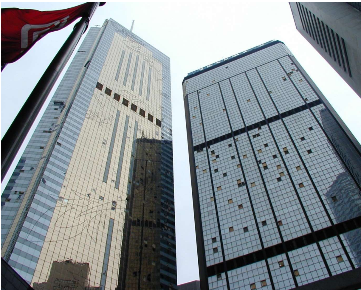
Figure 14 - Hong Kong, 1999. Typhoon York damaged the curtain walls of many buildings in the Wan Chai area. Wind-borne debris caused the breakage of glazed panels in the highest tall building floors (photo courtesy of Joe Khoury).
