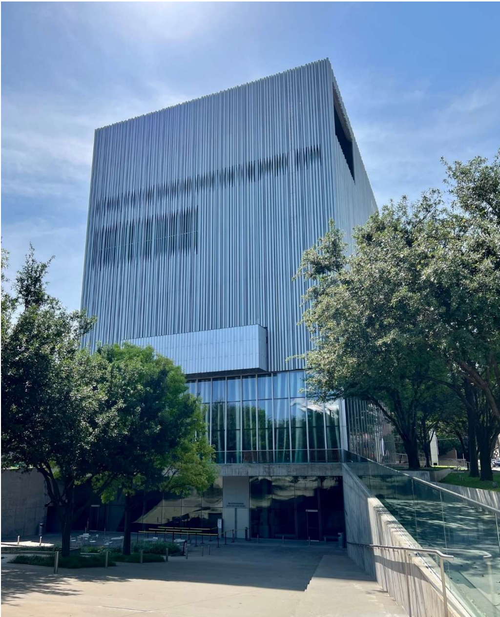
Figure 64 - Dallas, Dee and Charles Wyle Theatre. The building skin presents acoustic performances to address the requirements of the theatre. Moreover, some of the panels can be opened to let the actors enter the stage from alternative building entrances. 466 extruded aluminium tubes form the external cladding of the building, and these were designed to meet deflection criteria without the need of a subframe. A motorized black-out system shades the interior when necessary. A similar solution can be designed to withstand the impact of projectiles without requiring all the impact resistance to be on the glazed surface.
