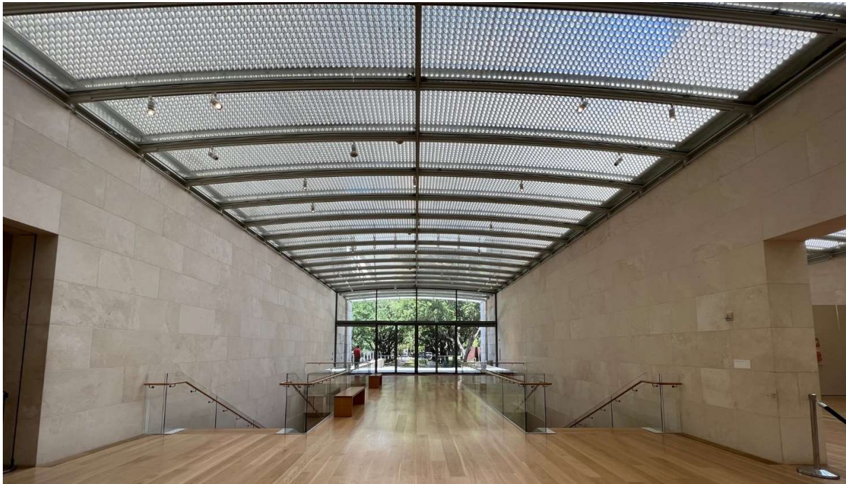
Figure 59 - Dallas, Nasher Sculpture Centre, designed by Arch. Renzo Piano, completed in 2003, interior view. The building roof has been designed to allow natural light to penetrate within the internal space of the museum. To reach the desired features, the building roof has been realized as a double-skin. To avoid glare, reflections in the exhibition area and to a porous external aluminium skin.
